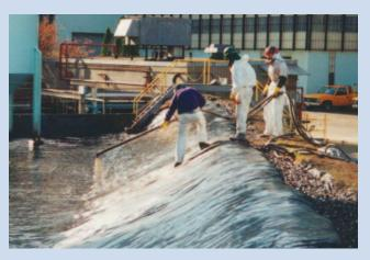
Due to its unique elastomeric qualities, CIM can bridge cracks and gaps in dissimilar materials such as steel, concrete and earth, even under extremely harsh environmental conditions.
